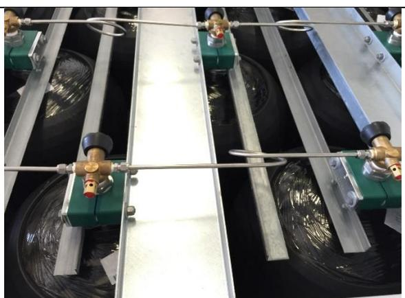
Detail of pipe connection of composite cylinders
