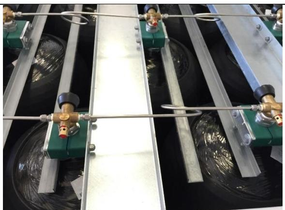
Detail of pipe connection of composite cylinders
